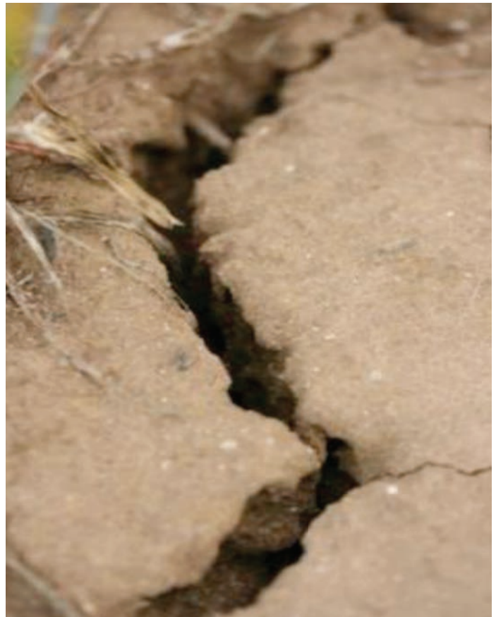
Clay soil with cracks
